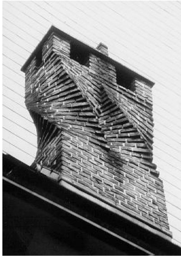
Figure 9: Screwed chimneys in Hamburg, Germany
