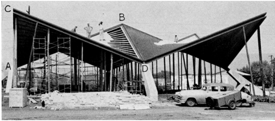
Figure 6: An application of hyperbolic paraboloid (H-P shell) [1]
