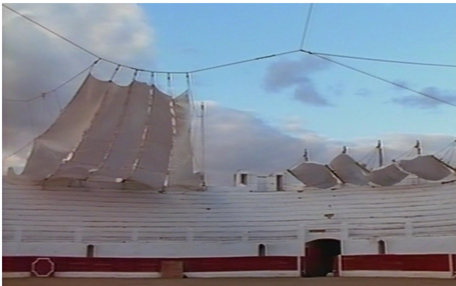
Figure 12: Two possible models for the velarium . The rope-supports are more vulnerable to high winds, while the masts are shorter but can be retracted in hostile weather (WGBH 2006).
