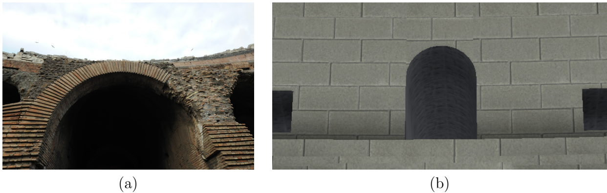
Figure 26: A comparison between one of the vomitoria in the Colosseum (a) shows that it does not have the attic overhead, as in the corresponding structure in the model (b).
