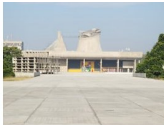
Assembly Hall (Chandigarh)
