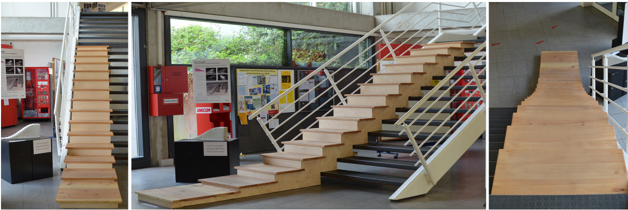
Figure 18: Installation of the walk-in sinus staircase in the faculty building: view from below, from the side, and from above.
